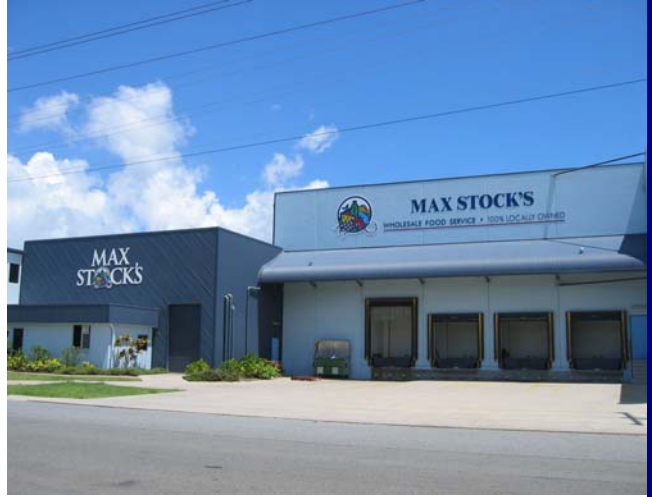
Commercial Facility - Cairns
